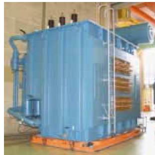
160 MVA steel EAF Transformer. Internal closure.
